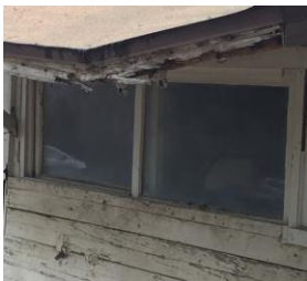
Close-up of deteriorated rafter tails on the shed. (photo by Joe Catalano)
