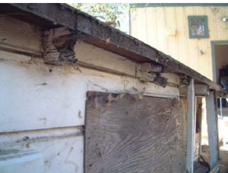
Close-up of deteriorated rafter tails on the shed. (photo by Joe Catalano)
