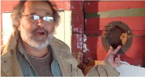
Joe Catalano points out a buried kitchen flue hole in Richardson House, discovered when the gypsum board was being removed.
